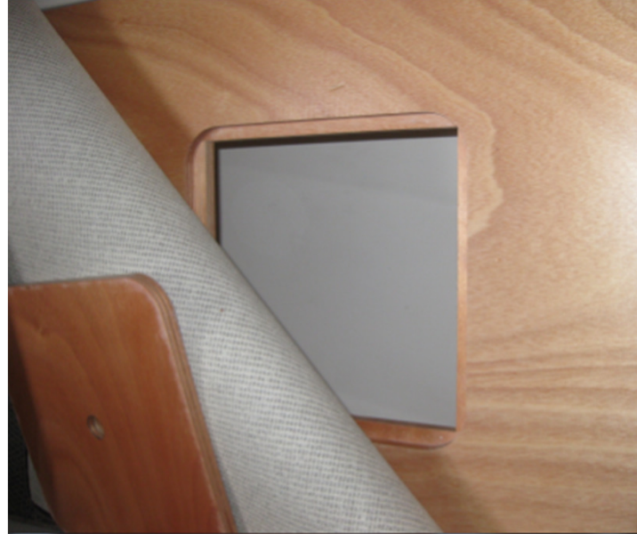
Pict.21. Under floor below the stairs
